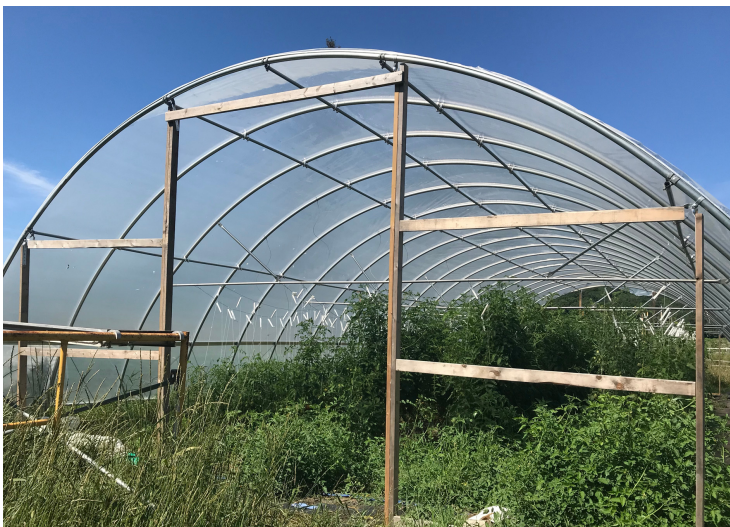
End wall framing on larger hoop house
